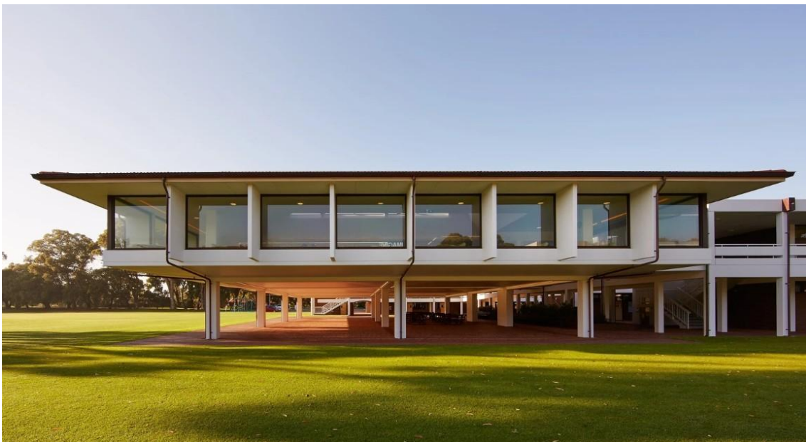
St Mary's Anglican Girls' School Library (Ferguson Architects website 2024)
